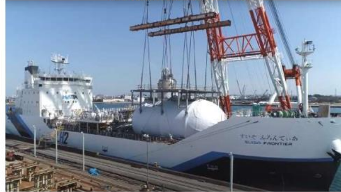
Cargo Tank Installation (7 March 2020) at KHI Harima Works
