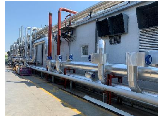
Fig. Connection to common rail cold
