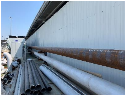
Fig. Connection adiabatic chiller
