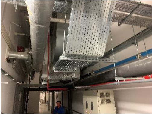
Fig. Technical mezzanine (cable par prepared, main cables placed
