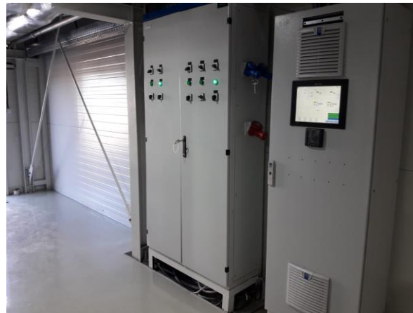
Fig. CHP room – electrical control
