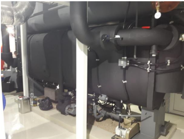
Fig. CHP room – absorber chillers
