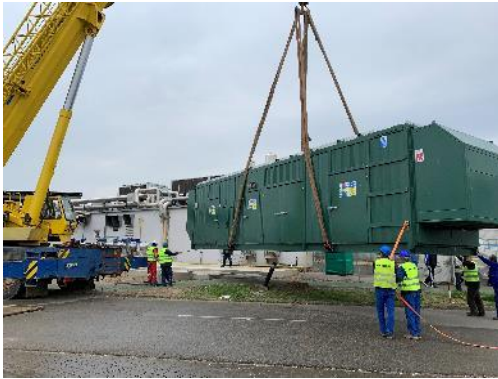
Fig. Generator 50T in air
