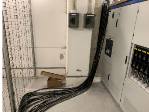
Fig. Technical mezzanine (cable par prepared, main cables placed
