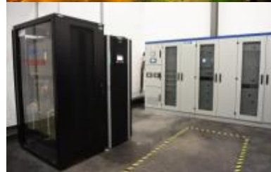
Webaxys datacenter with xStorage Buildings 40kW scalable storage Le Havre, France
